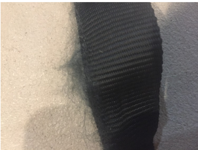
Webbing showing signs of heavy abrasion
